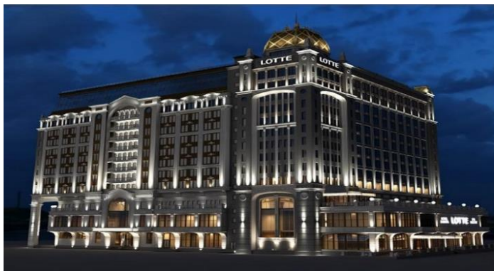
Lotte Hotel 4 pcs 1600kva 11/0.4kv
